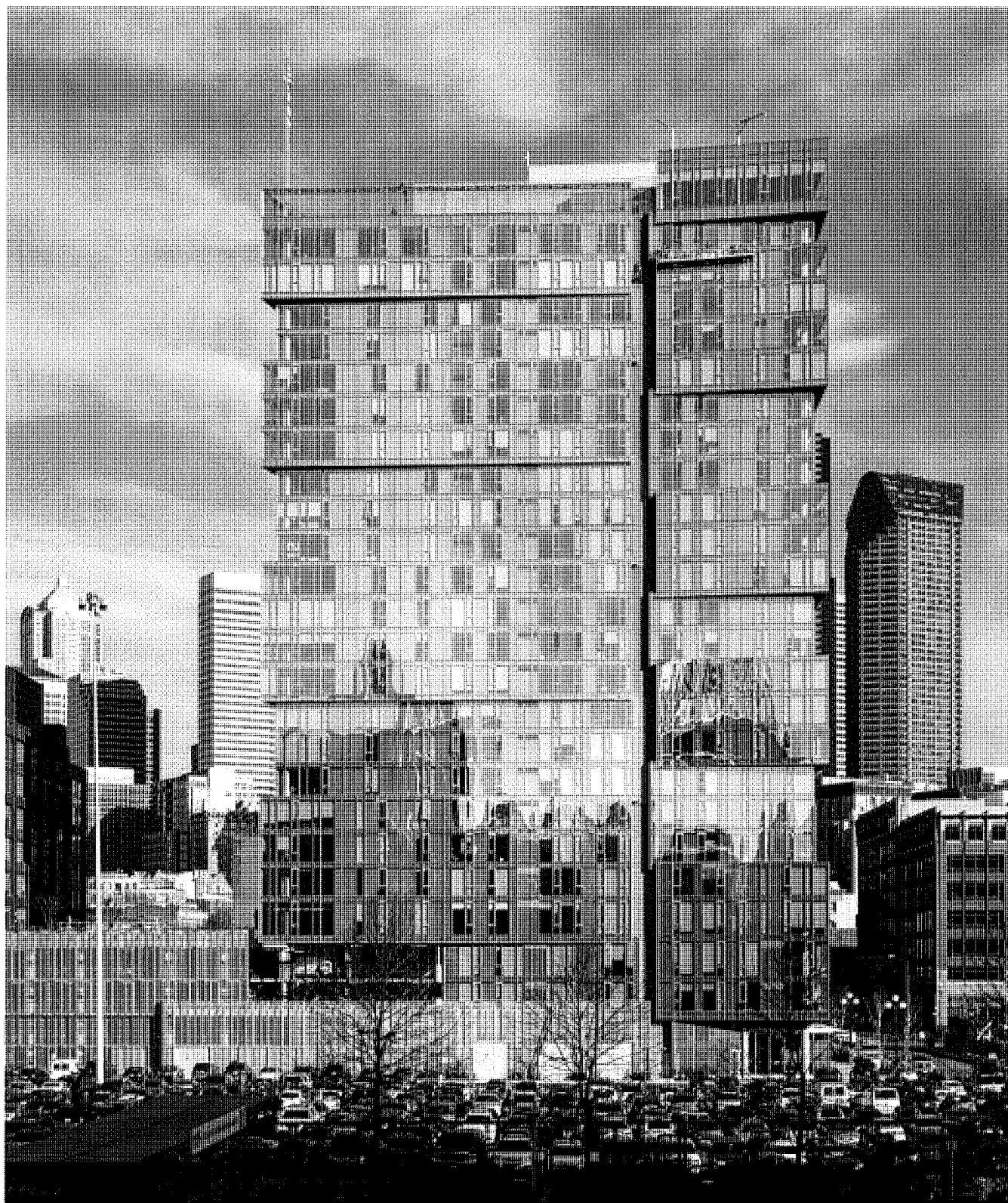
The Wave apartment building is part of the Stadium Place hotel, apartment and office project north of CenturyLink Field in Seattle, financed by EB-5 money. (Mike Siegel / The Seattle Times)
