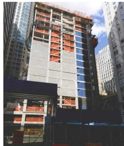
In Construction ("Phase I"): April 22, 2013
