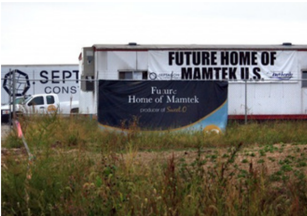
MAMTEK SUCROSE PLANT
