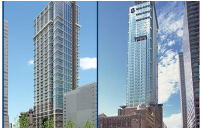
MIXED-PURPOSE 50 STORY TOWER DENVER, COLORADO
