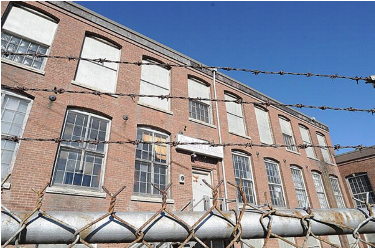
Whittenton Mills in Taunton, MA, site of an EB-5-funded redevelopment
