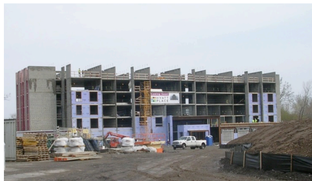
Figure 9. The Hyatt Place Hotel under construction in May 2014
